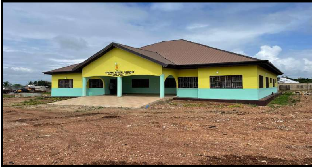
Figure 3: Commissioned and Operationalized 1 No. CHPS compound at Asuotiano (DACF)
